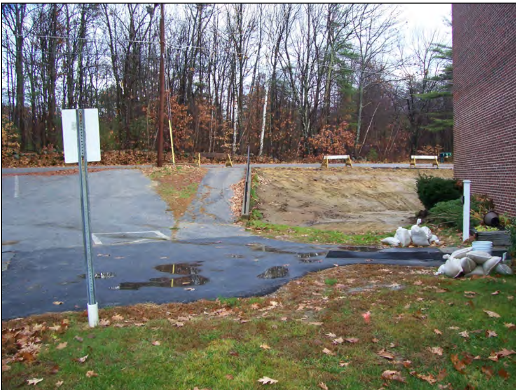
Civil Photo 8: Paved ramp connecting parking lots, looking north.
