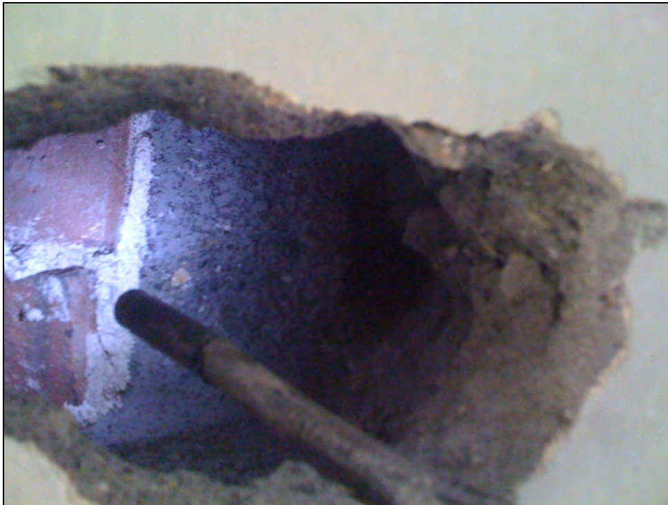
Core of CMU block; visible brick is tie to brick veneer.
