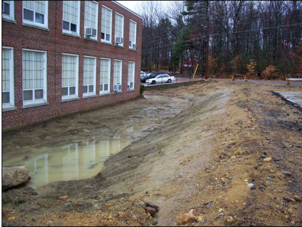
Civil Photo 15: Slope between building and upper parking lot.
