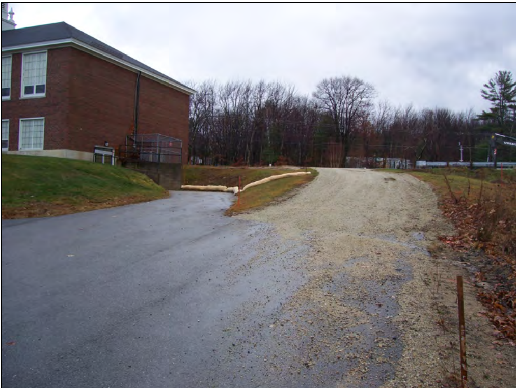
Civil Photo 10: Gravel drive from upper lot to driveway intersecting Route 9.
