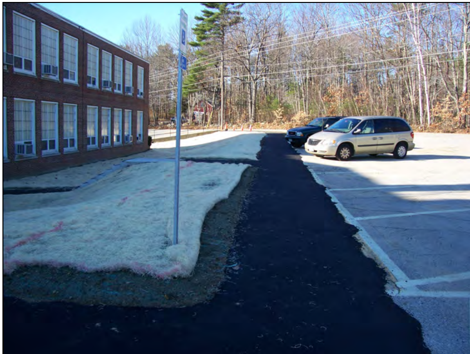
Civil Photo 18: New sidewalk at upper lot, looking west.
