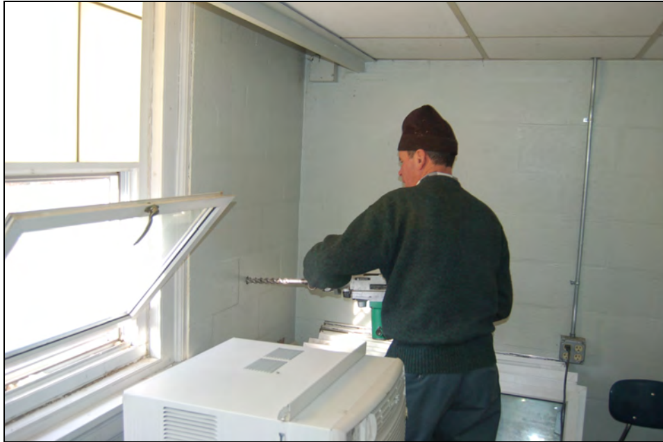
Drilling holes through the CMU.
