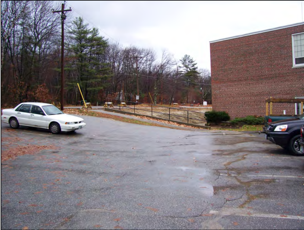
Civil Photo 7: Paved ramp connecting parking lots, looking northeast.
