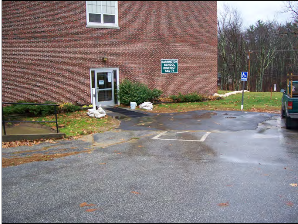
Civil Photo 5: Accessible space at lower parking lot and accessible building entrance.
