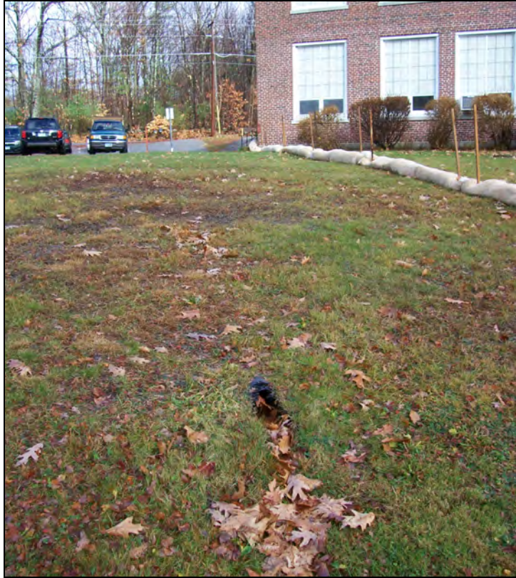
Civil Photo 13: Existing outlet from drop inlet.
