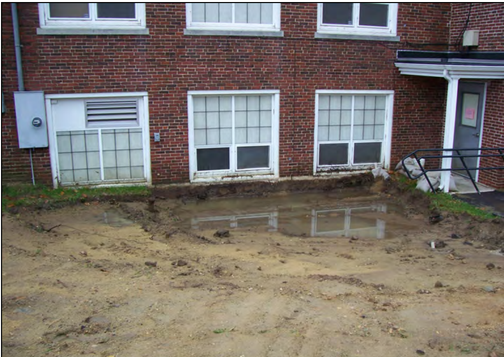
Civil Photo 12: Finished grade at windows and door pad.
