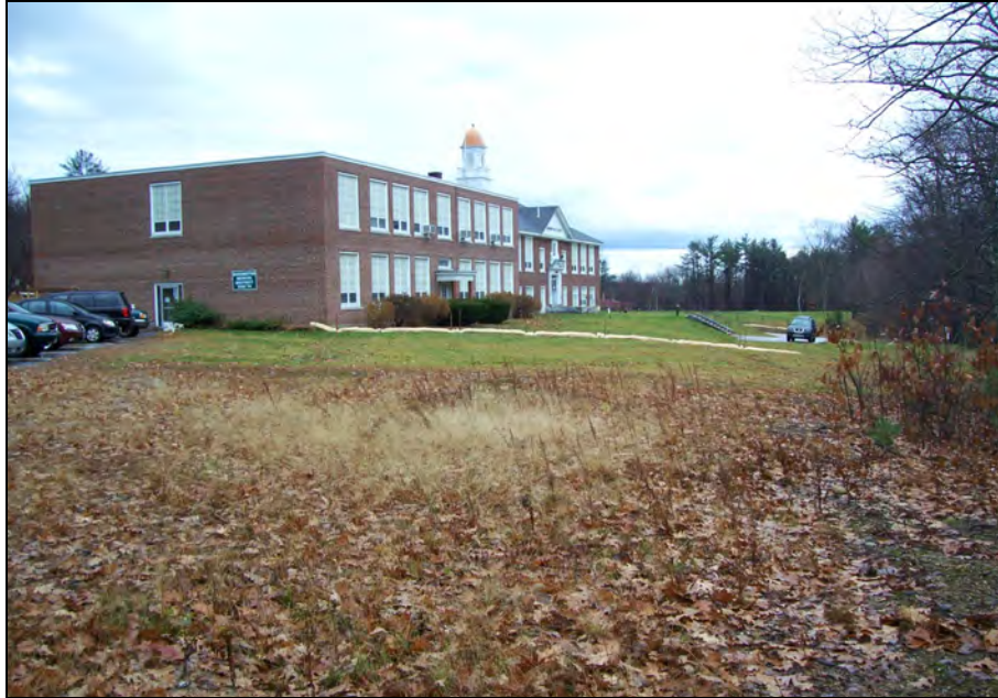
Civil Photo 1: Grassy expanse down slope from lower parking lot, looking east.
