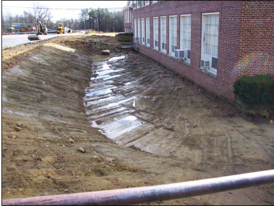
Civil Photo 17: Drainage improvements in progress (fall 2010).
