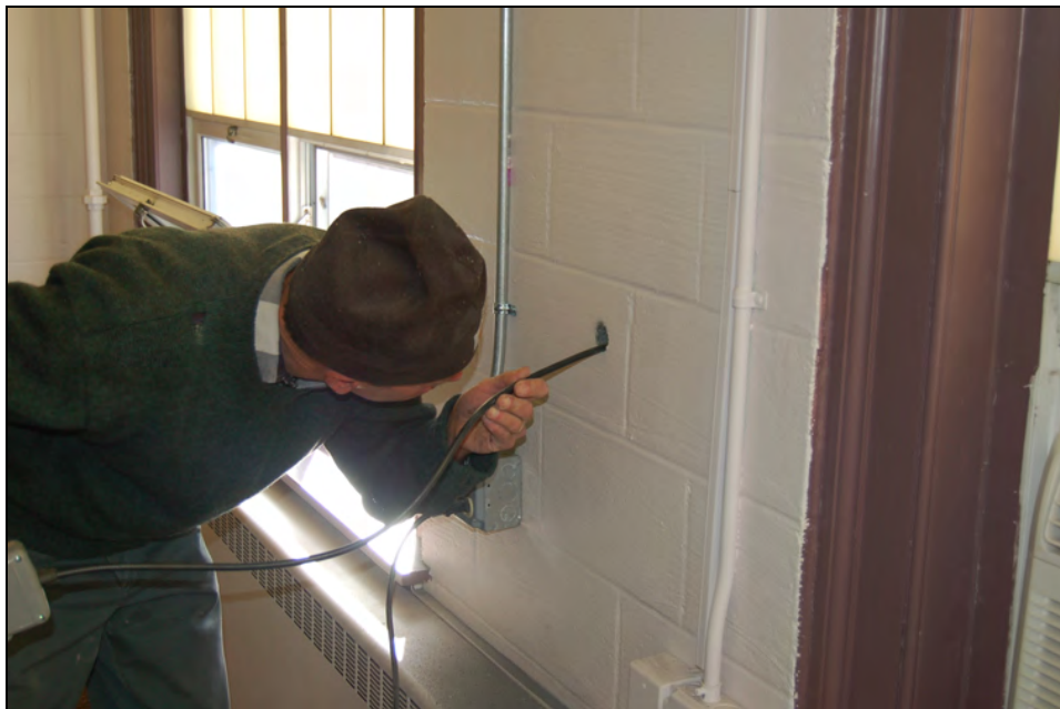
Using a camera probe to view the wall cavity.
