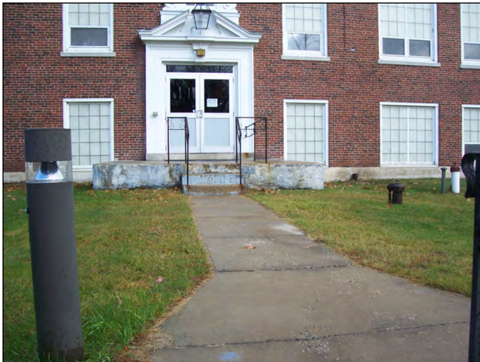
Civil Photo 14: Existing stairs at employee entrance.
